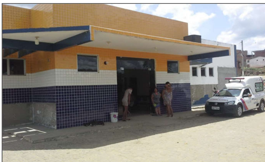
Figura 21 – Gandu: Hospital João Assis
